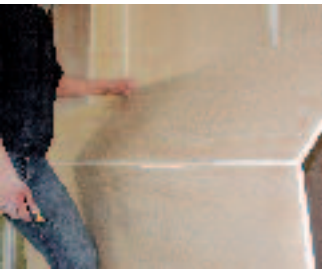
3. Board has to be cut from the decor side.
